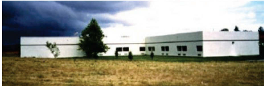
Figure D-1 Templeton Hospital before the 2003 San Simeon earthquake; view looking southwest with north wing shown on the right (CSMIP, 2015).
