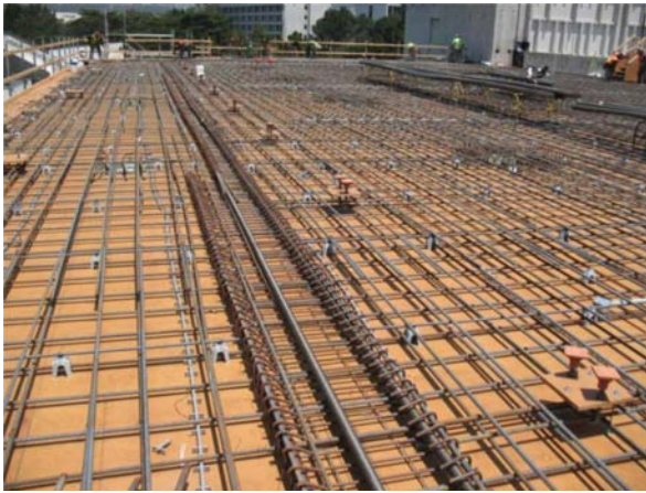
Figure 9-2 – A long collector with confinement reinforcement.
