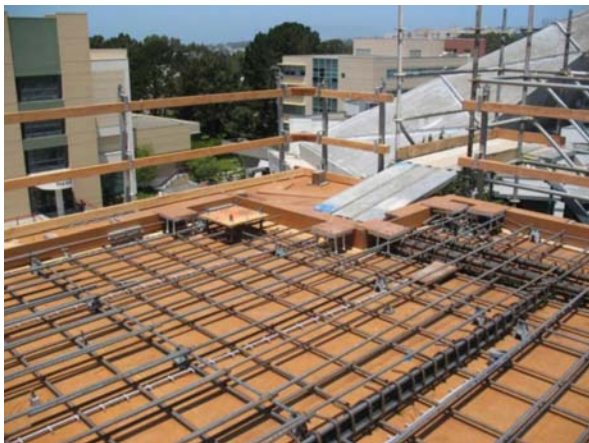
Figure 9-3 – Confinement of a collector.
