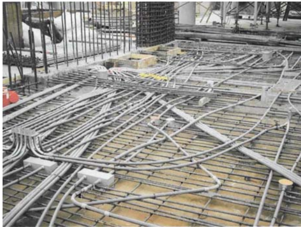
Figure 9-5 – Embedded conduit.
