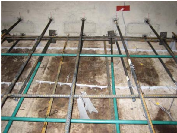
Figure 9-4 – Form savers for dowel anchorage.
