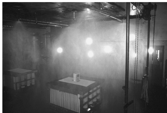
FIGURE F.3(b) Water Mist Discharge.
