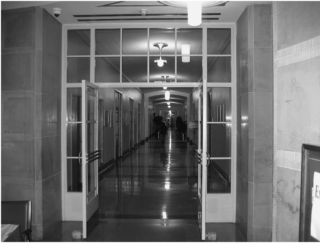
FIGURE F.2(b) Rated Glass Corridor Doors in Normal Position.
