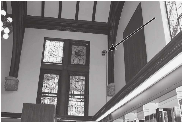
FIGURE F.4(c) Linear Beam Smoke Detector.
