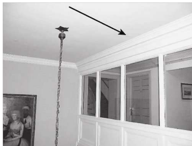
FIGURE F.3(a) Sprinklers to Maintain Glass Cooling.
